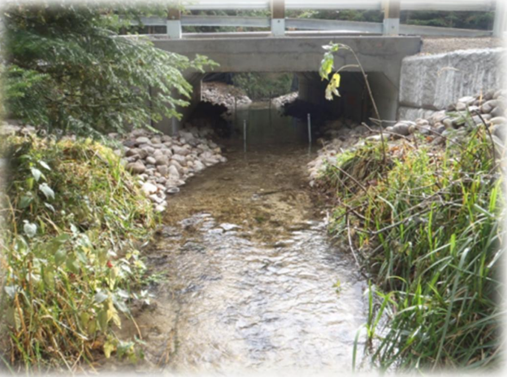
Replaced with the Barefoot Box Culvert™
