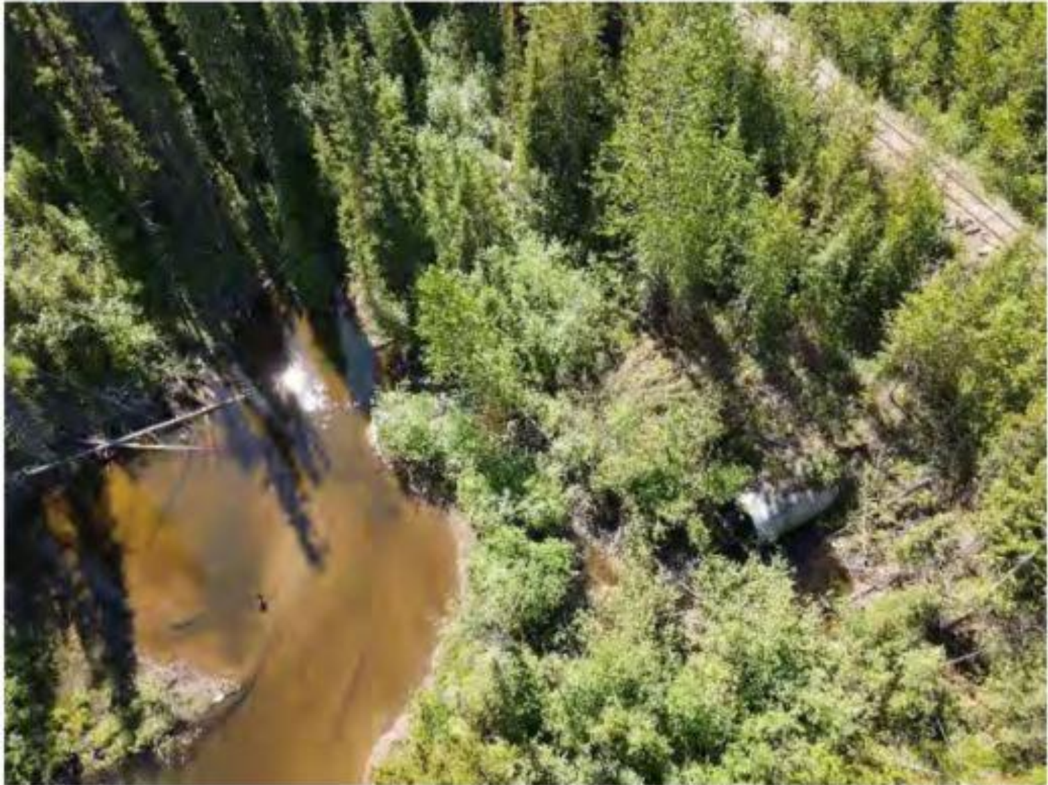
Figure 1-5: Aerial view of channel flowing into culvert inlet
