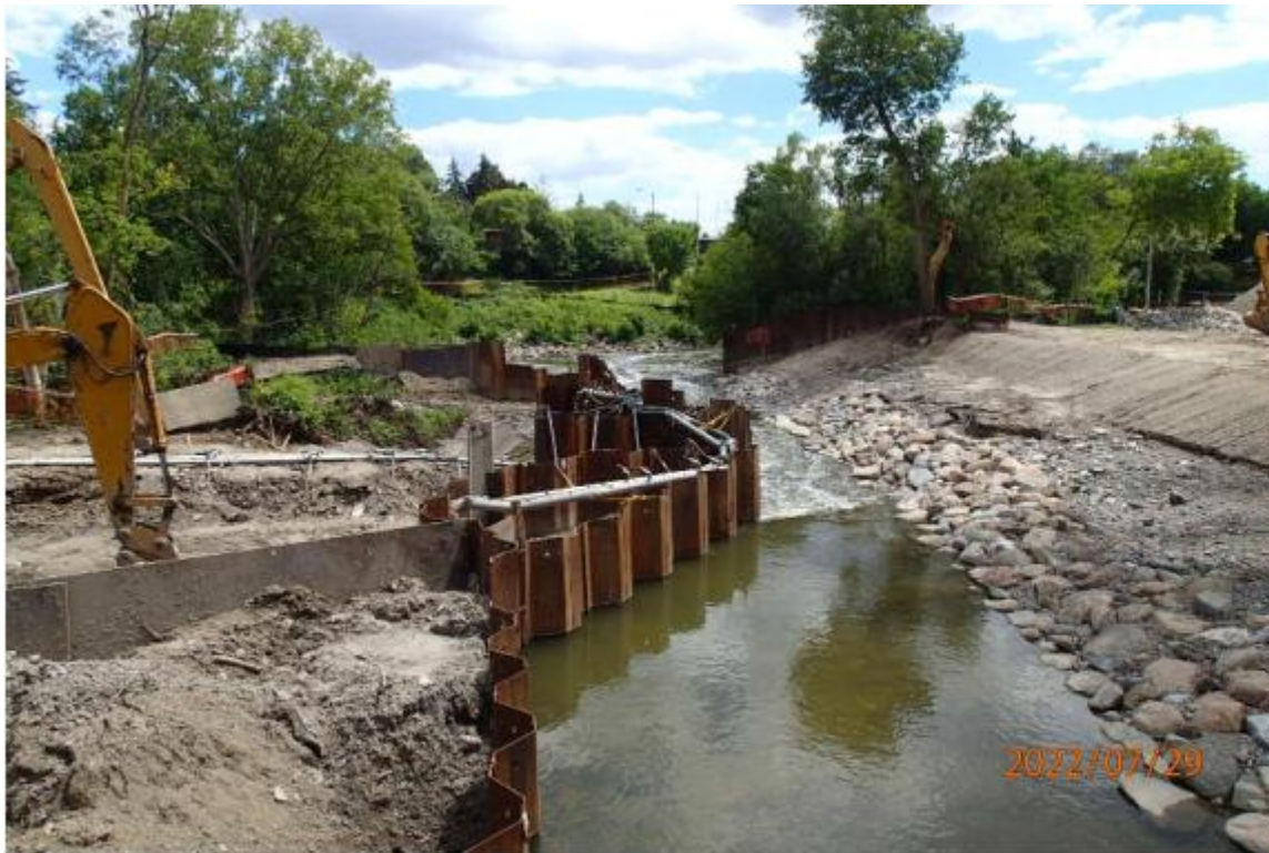
Picture 27: Site conditions, south of bridge.
