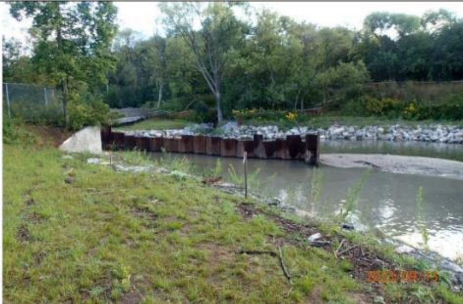
Picture 13: Cofferdam sheet pile removal.
