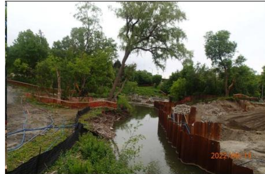
Picture 6: Leaning tree removal.
