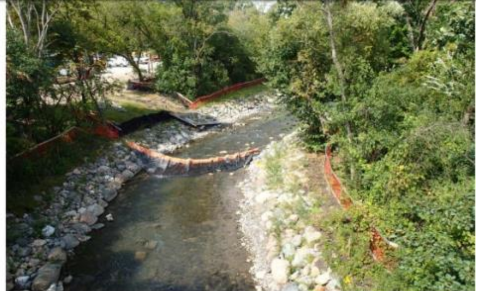
Picture 14: Cofferdam, silt curtain placement.
