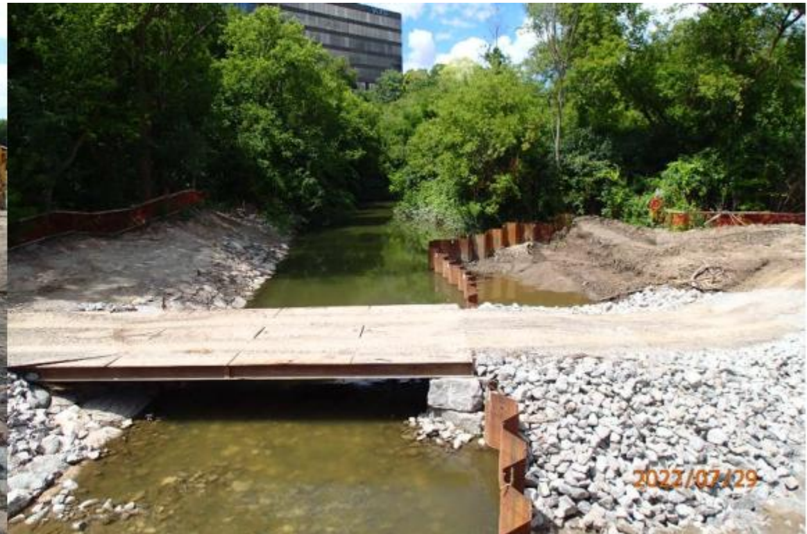
Picture 28: Site conditions, north of pedestrian bridge.
