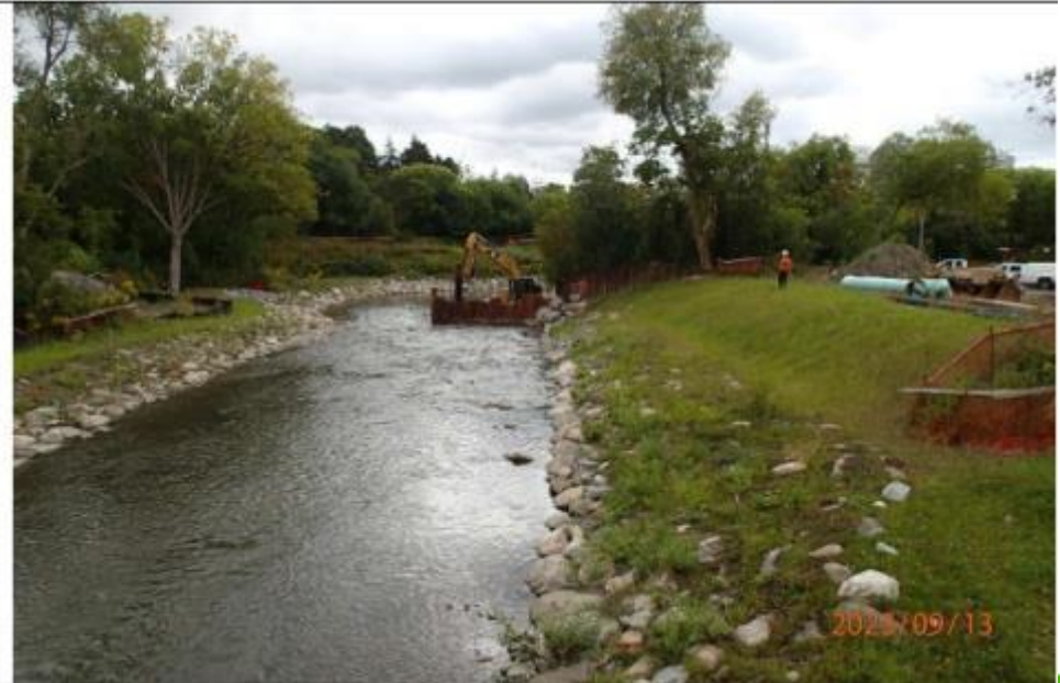
Picture 14: Cofferdam, silt curtain placement.
