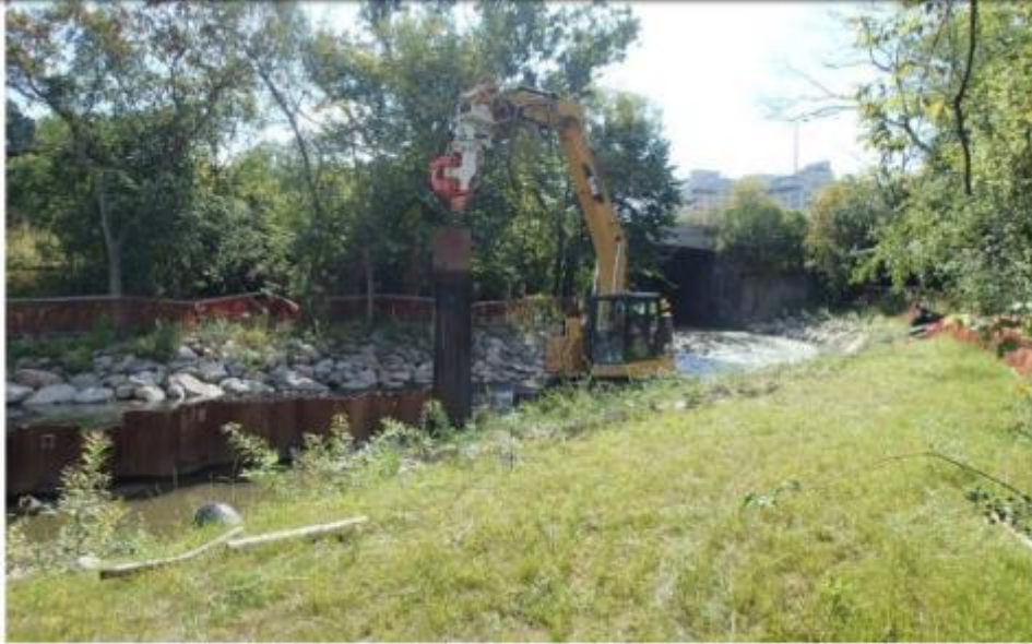
Picture 13: Cofferdam sheet pile removal.
