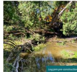
Log jam pre-construction
