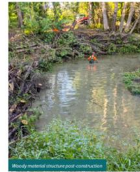
Woody material structure post-construction
