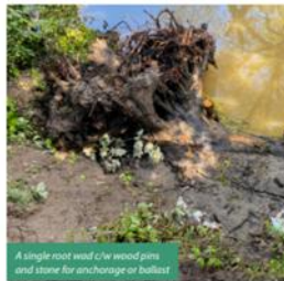
A single root wad with wood pins and stone for anchorage or ballast
